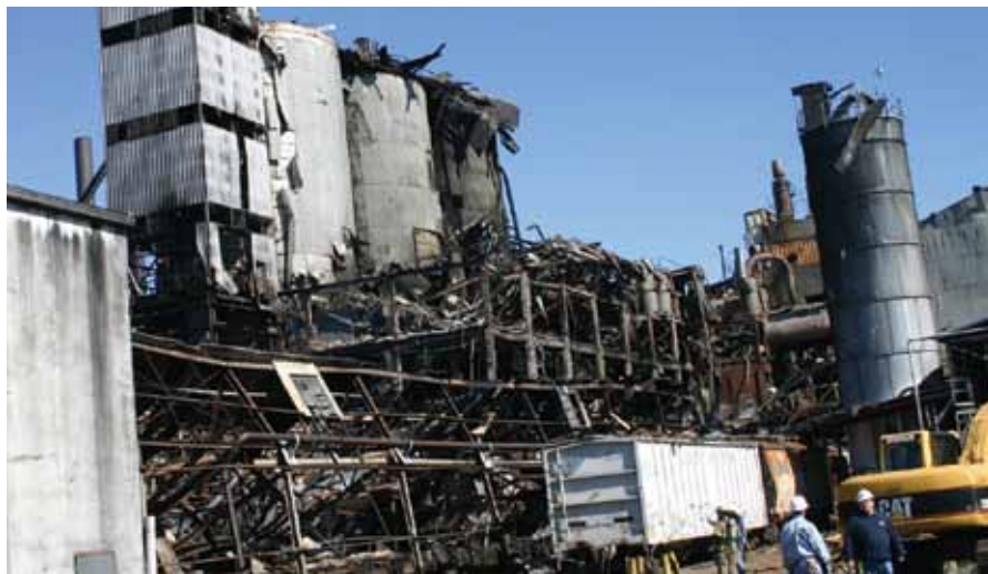
Investigators and firefighters at the site of the explosion and fire at the Imperial Sugar Refinery in Port Wentworth, Ga.
